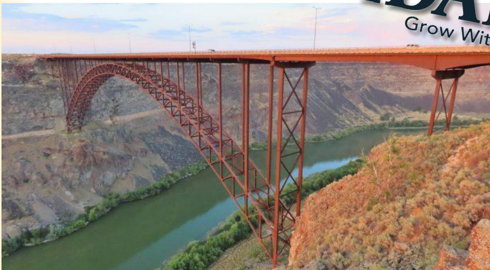
Perrine Bridge // Truss Arch. Idaho's famous Perrine Bridge is a four-lane truss arch span on U.S. 93 over the Snake River in Twin Falls.
